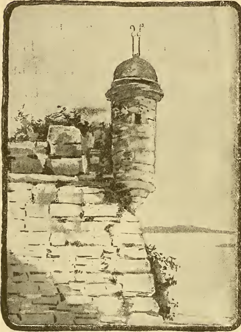
THE TOWER OF THE FORT.
